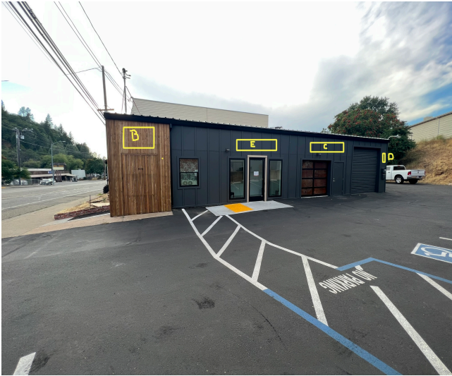
Eastern side wall facing parking lot.
